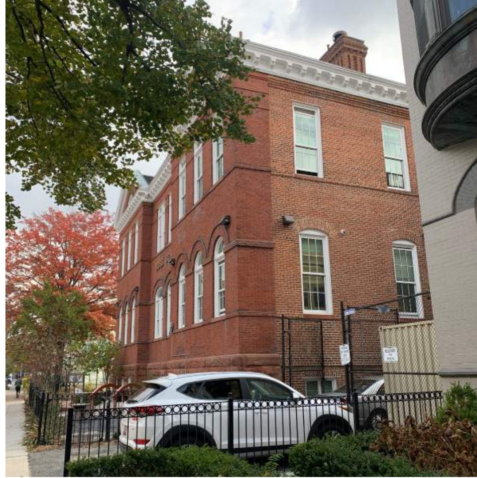
View D: building NW corner, view from R St
